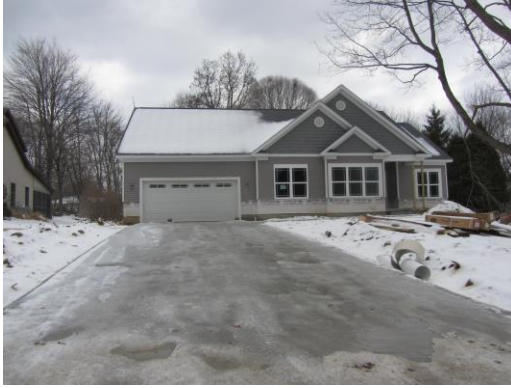
New House Construction on Stanley Road former razed lot
